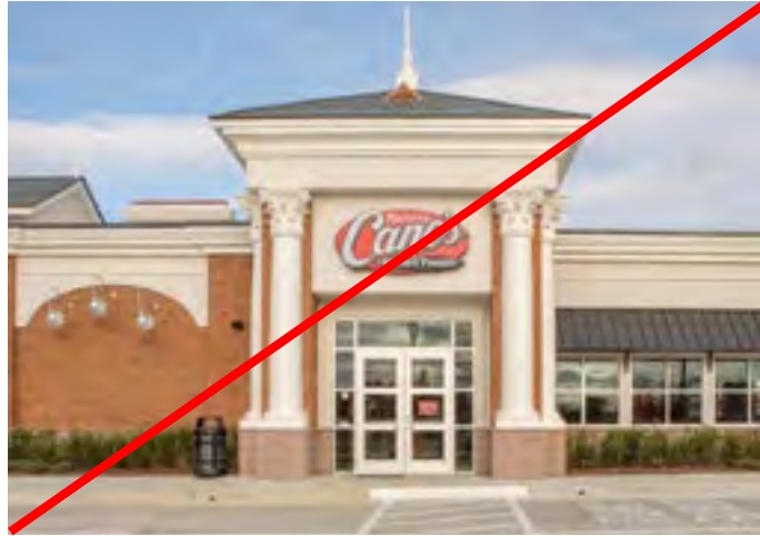
Fiberglass classical ornamentation and poorly applied.
