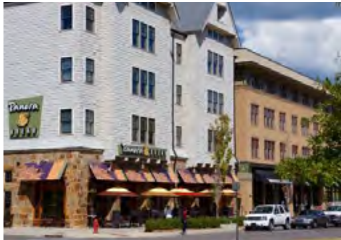
Heavy stone used below lighter siding material.
