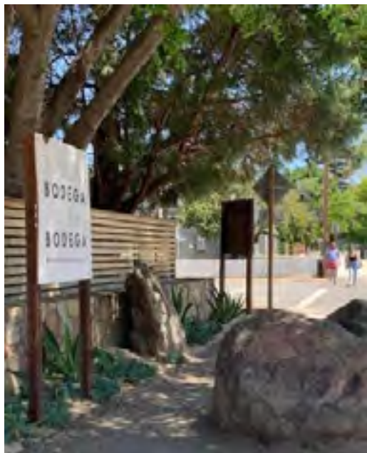
Landscaped retaining wall and fence.
