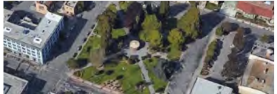
PHOTO CAPTION —Aerial view of Watsonville City Plaza
