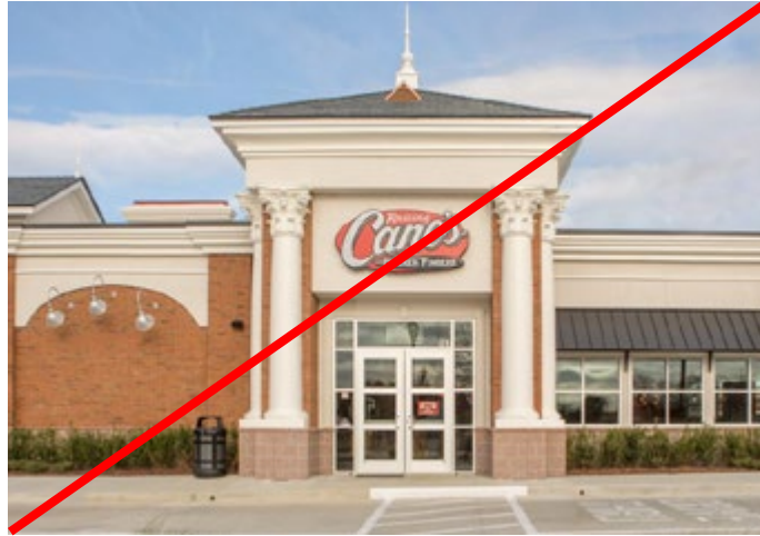
Fiberglass classical ornamentation and poorly applied.
