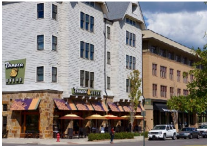
Heavy stone used below lighter siding material.
