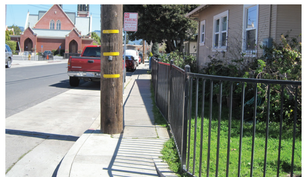
Figure 5 | Utility Pole Narrowing Sidewalk on Ford Street
