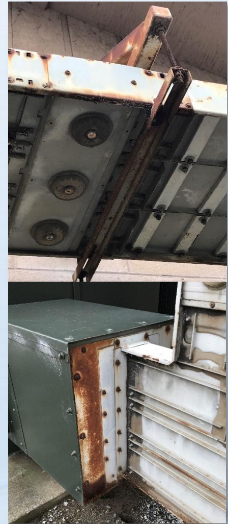
Significant Corrosion (Transformer Busway)
