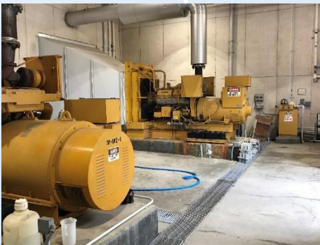
Standby Generators in Energy Recovery Building
