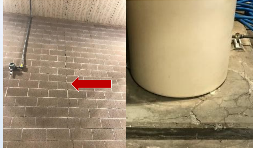
Repair Cracks/Spalling (Energy Recovery)
