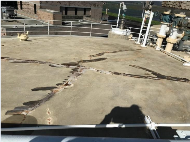
Repair Roof Cracks From Above (#2)
