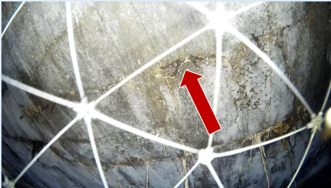
Repair Possible Roof Cracks From Interior (Drone Inspection of #2)
