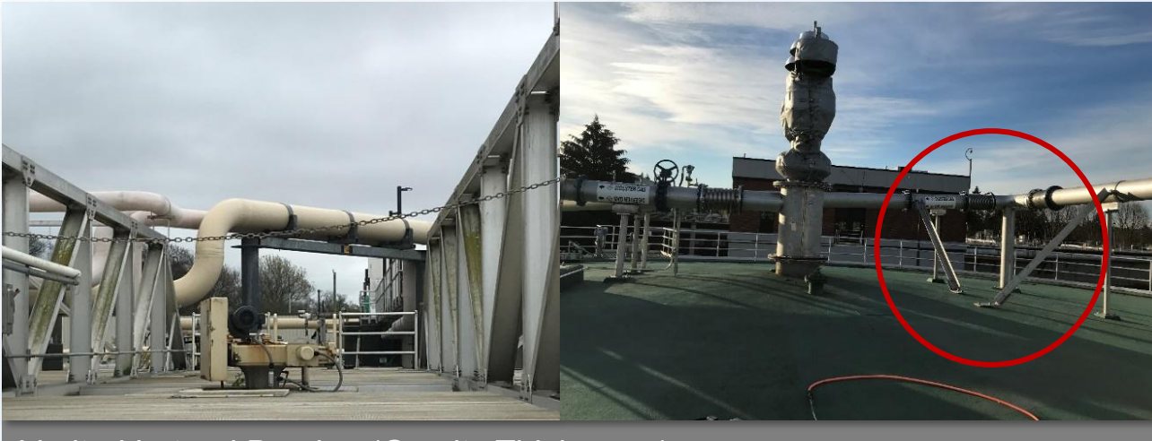
Limited Lateral Bracing (Gravity Thickeners)
