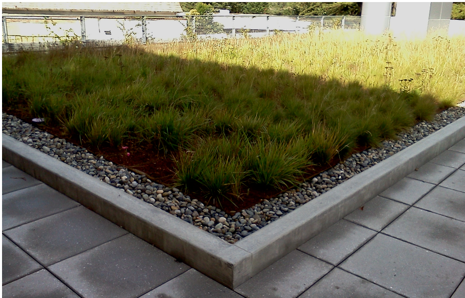
Figure 4.5 Concrete curb with vegetation-free zone. Green Roof Report, City of Watsonville CA
