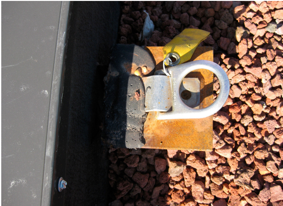
Figure 4.3 Hooks for safety equipment in the vegetation-free zone.
