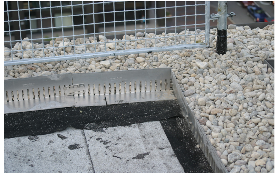
Figure 4.6 Metal edge restraint contains gravel in vegetation-free zone.
