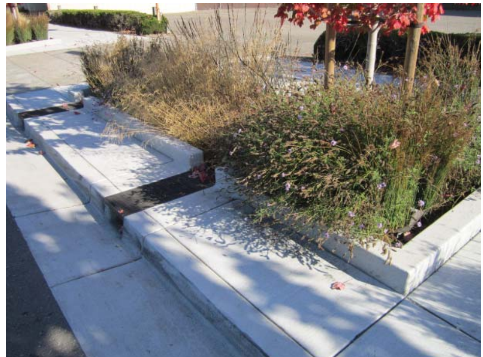
Street runoff flows through curb cuts into stormwater planters, El Cerrito, CA
