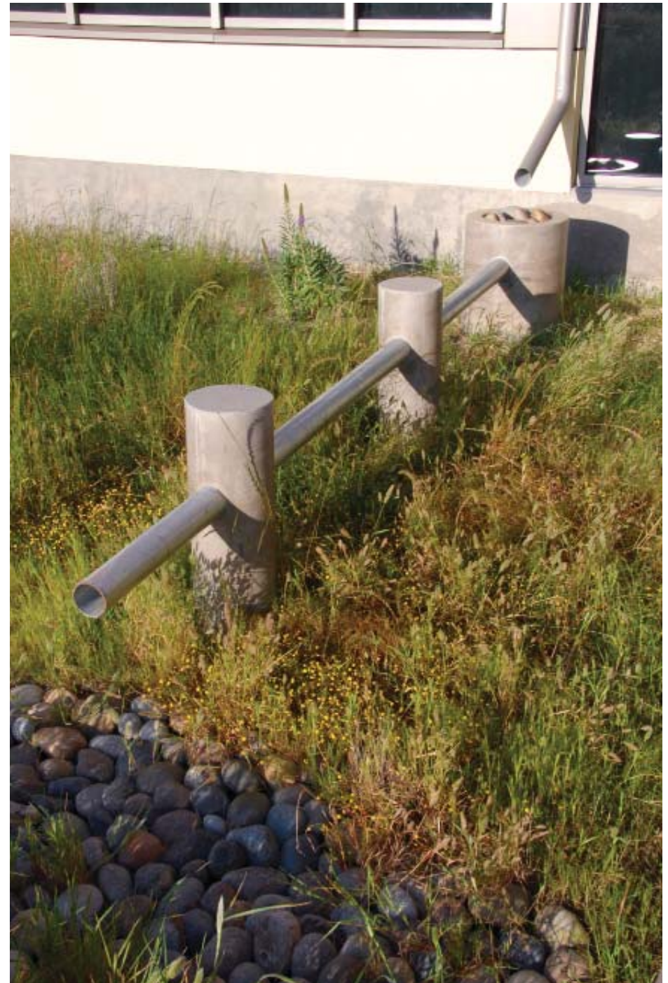
Rainwater funneled from the roof to a bioretention planting area at the Redwood Shores Library, Redwood City, CA
