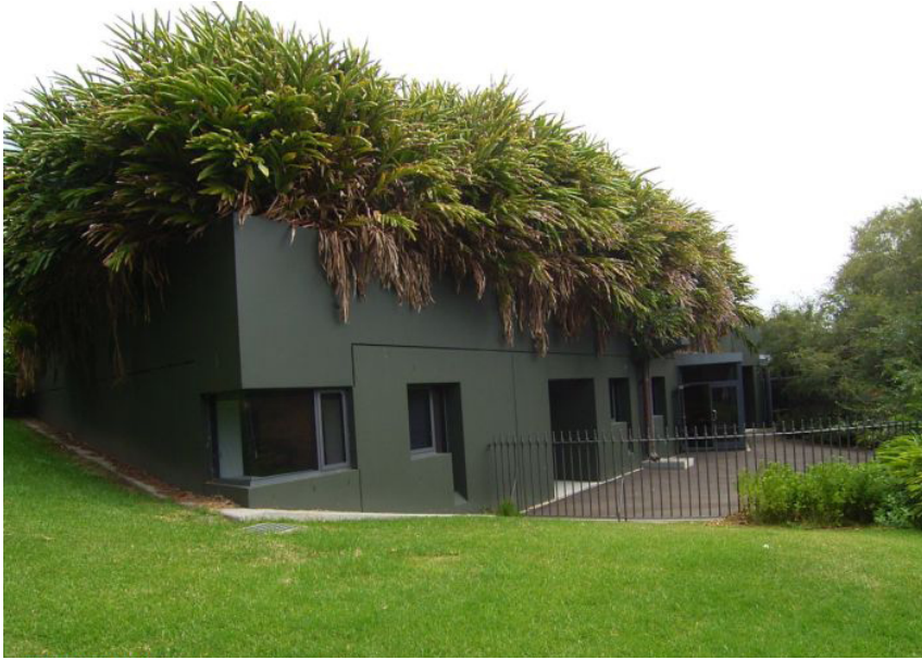
Figure 2.2 An example of an intensive living roof
