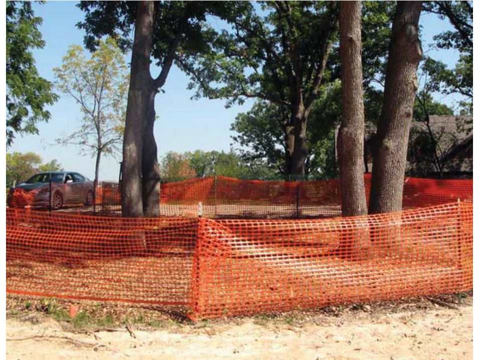
Tree protection fencing at a construction site
