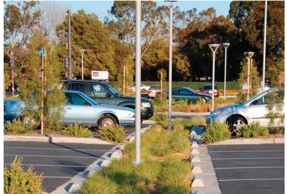
A vegetated swale filters stormwater at the Redwood Shore Library in Redwood City, CA.
