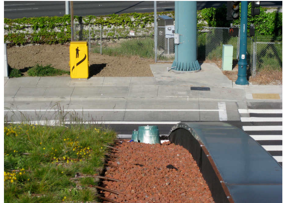
Figure 4.4 Vegetation-free zone at parapet, with irrigation boxes showing.
